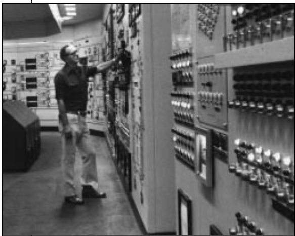
Simulated control rooms are used to train nuclear power plant operators to be prepared for emergencies.
