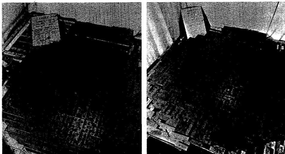
*Tenth layer of graphite blocks containing pseudospheres of black and brown uranium oxide. The brown briquets, slightly richer in uranium, were concentrated in the central area. In the foreground and on either side are cavities filled with graphite, now presumed to have been an expedient measure dictated by shortage of fuel and, possibly, a last minute change in the lattice arrangement. On the right is the 19th layer of graphite covering layer 18 containing slugs of uranium oxide.*
