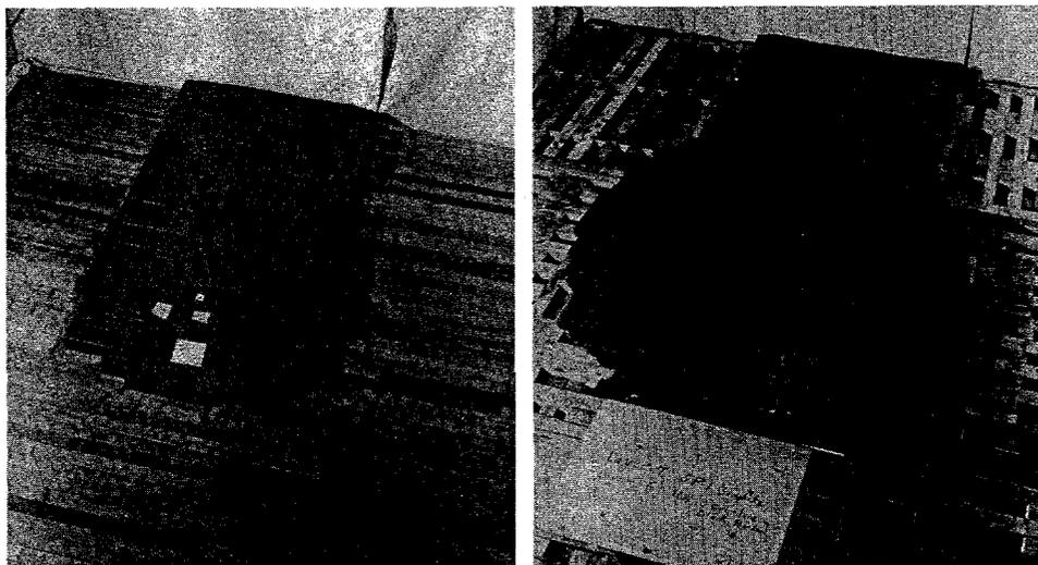
*Graphite layers form the base of the pile, left. On the right is the 7th layer of graphite and edges of 6th layer containing 3/4-inch pseudospheres of black uranium oxide. Beginning with layer 6, alternate courses of graphite containing uranium metal and/or uranium oxide fuel were separated by layers of solid graphite blocks.*
